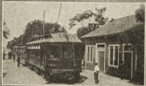
NORTHERN ELECTRIC DEPOT
