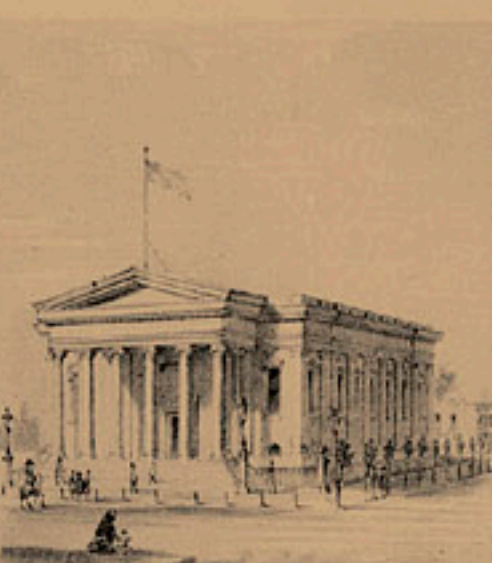
County Court House - (now used as State Capitol)
