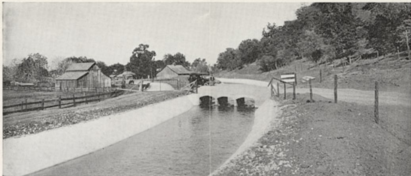
FROM CLEAR LAKE WATER IS DISTRIBUTED THROUGH EIGHTY MILES OF CANALS AND TWO HUNDRED AND FORTY MILES OF LATERALS
